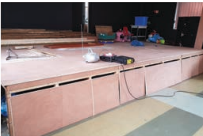
The old stage was in a bad condition so was replaced with a new plywood surface and improved storage.
